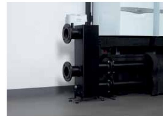
Low loss header in situ on boiler rig
