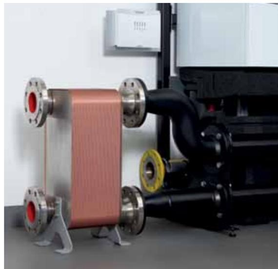
Low loss plate heat exchanger in situ on boiler rig
